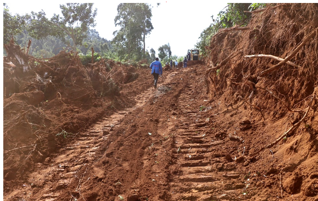
Road construction works in progress across the County
