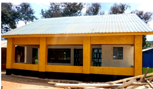
A newly completed ECDE classroom
