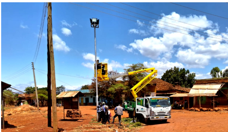
Energy department officers undertaking the security lights repairs
